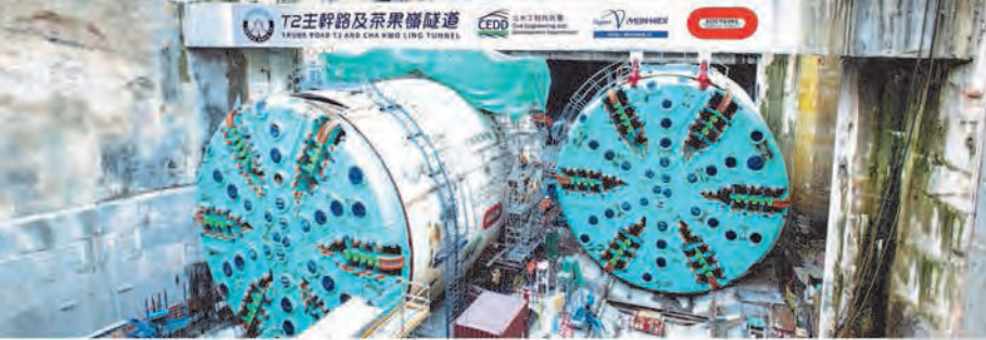
Kai Tak Development - Trunk Road T2
